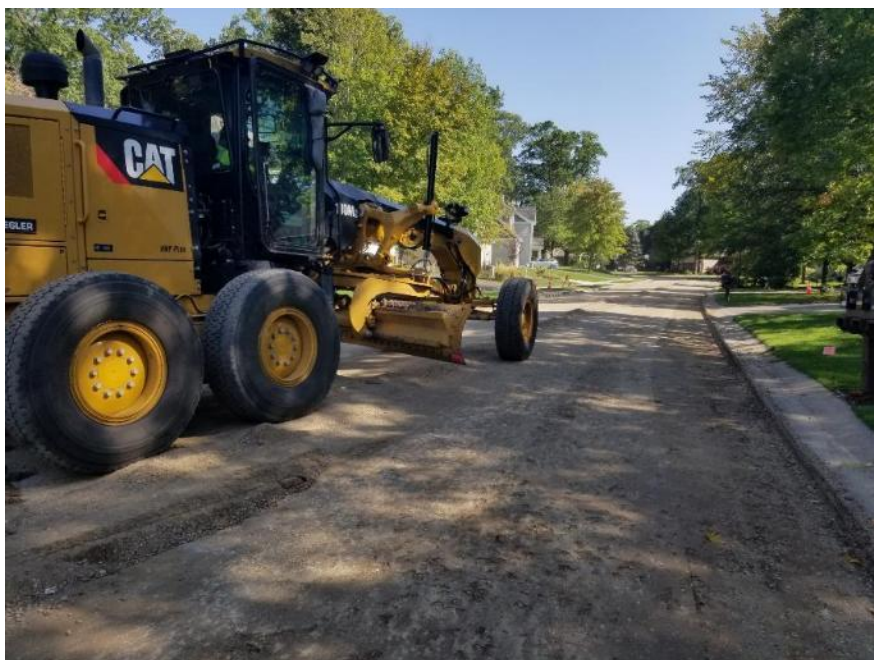
Pavement Removal and Grading
