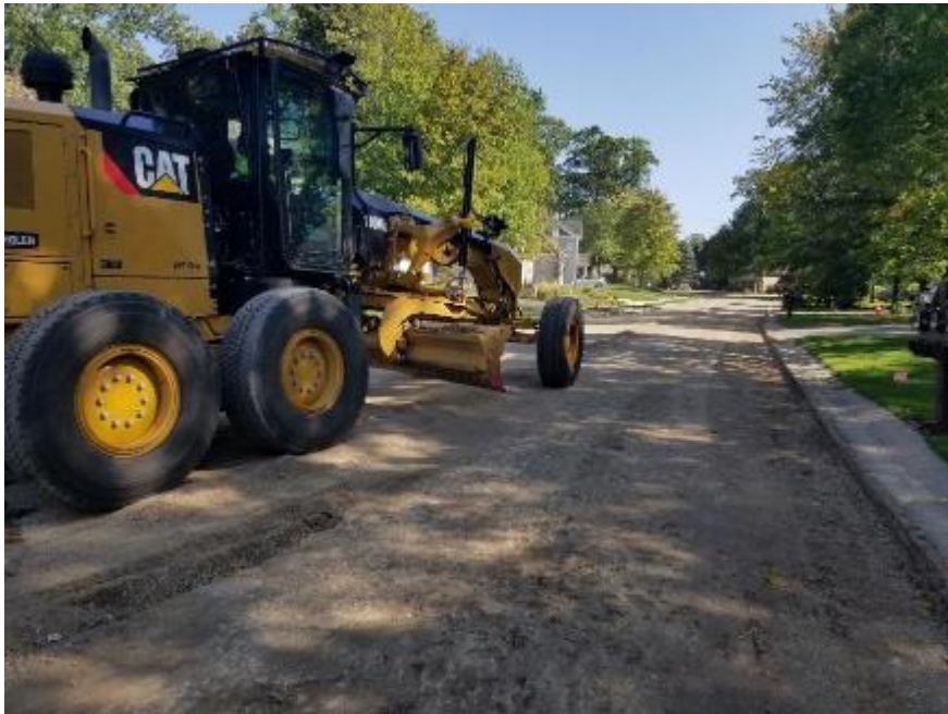
Pavement Removal and Grading
