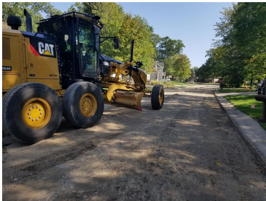
Pavement Removal and Grading
