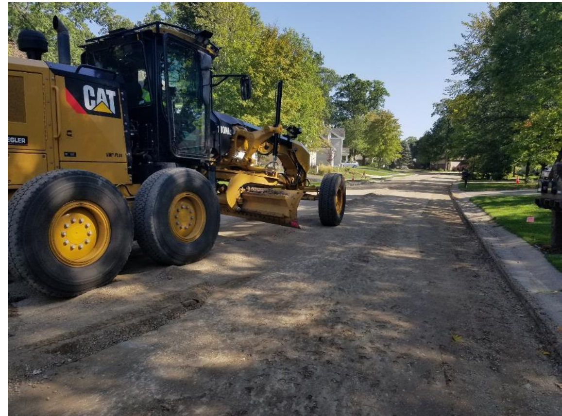
Pavement Removal and Grading
