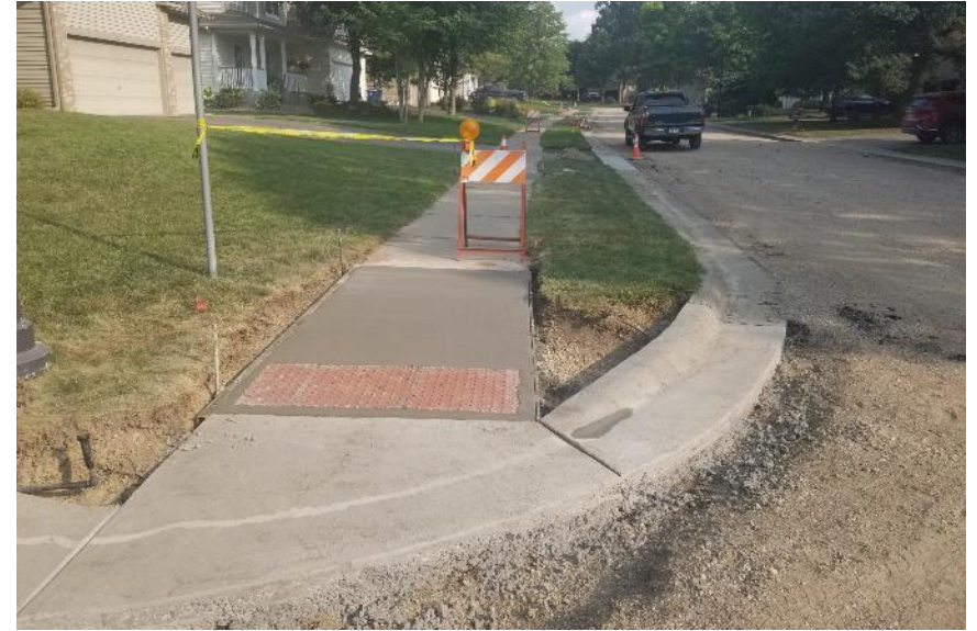
Sidewalk Pedestrian Ramp
