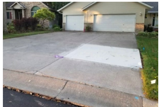
Figure 2. Example of concrete driveway replacement for curb stop repair.
