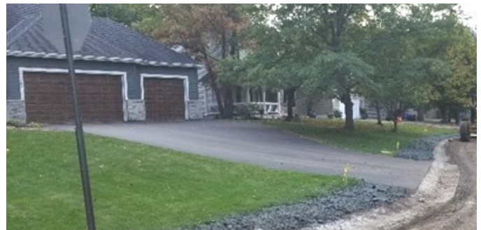
Figure 4. Example of complete bituminous driveway replacement where City reimbursed property owner for the portion of the driveway to be replaced with the project at the City project contractor price.
